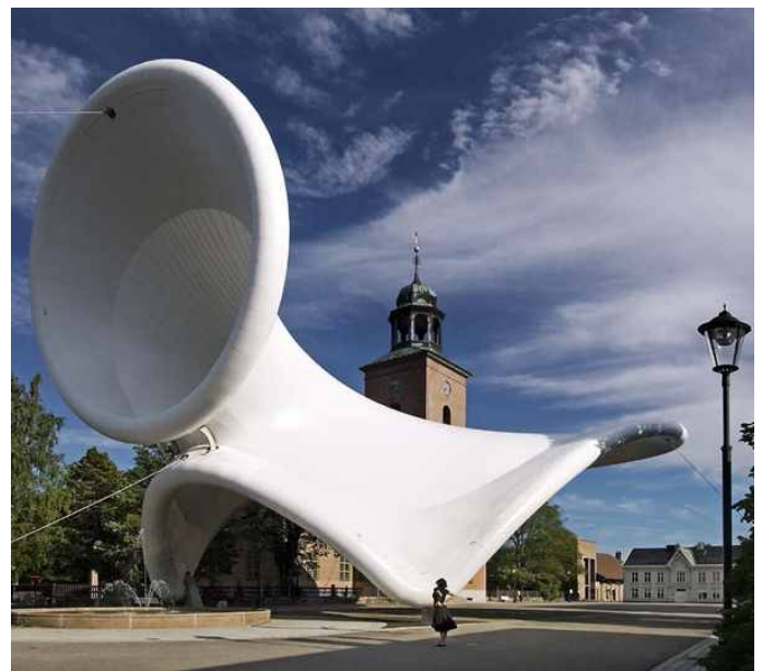
Fig. 28 | Tubaloon temporary concert hall (2006 Kongsberg, Norway) Snøhetta AS, Šorm TL
