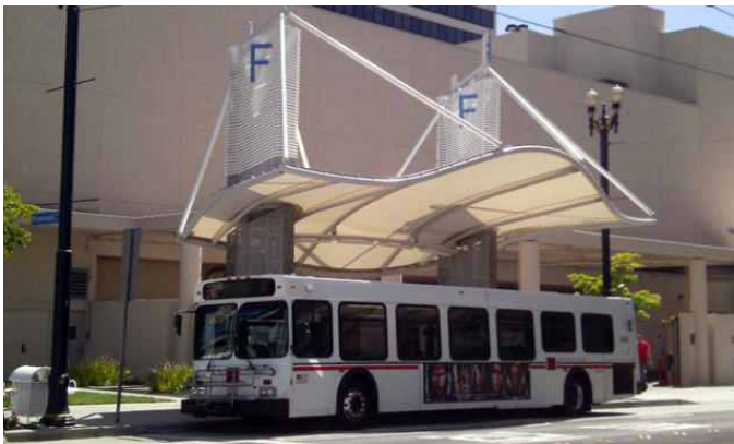
Fig. 11 | Bus stop shelter (2011 Long Beach, California, USA) MIG Arch., Birdair
